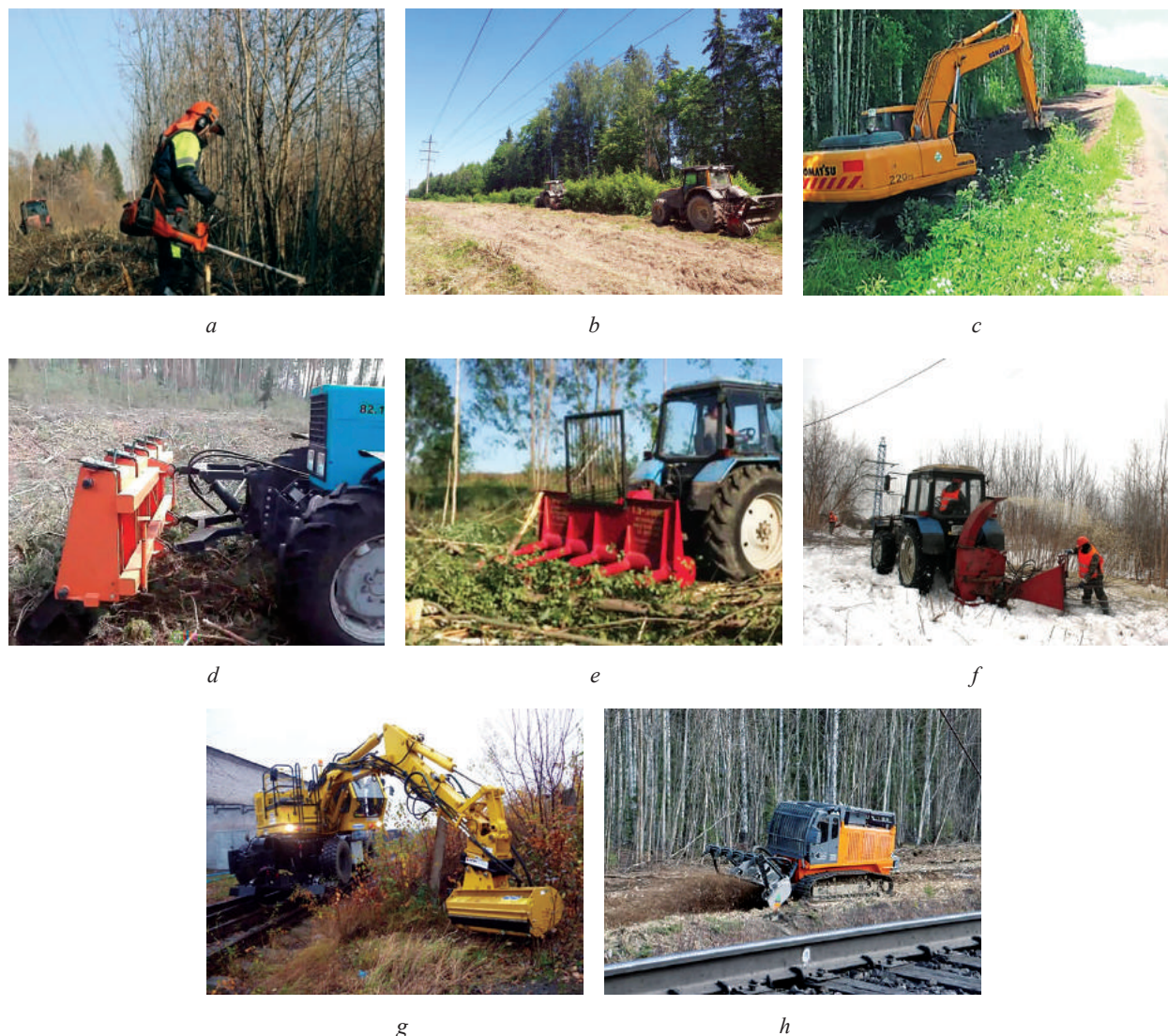
Fig. 2. Removal of unwanted trees and shrubs: a — in the security zone of the high-voltage line, Ryazan Region, April 2019; b — in the security zone of the high-voltage line, Moscow Region, June 2019; c — in the right of way of the road, Arkhangelsk Region, July 2016; d — forest rake EM 2200; e — forest rake GL-3000; f — in the security zone of the high-voltage line, Moscow region, February 2019; g — multifunction machine KGT-4RS with mulcher ORD; h — in the railway right of way, Republic of Buryatia, May 2020
